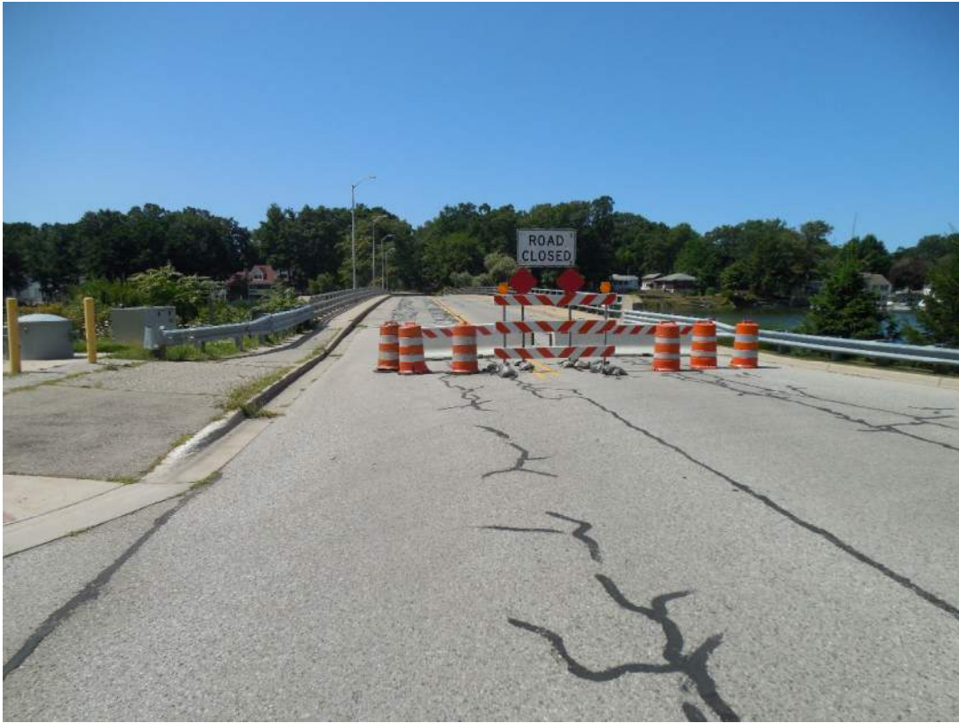
View of closure signage at north approach, looking south
