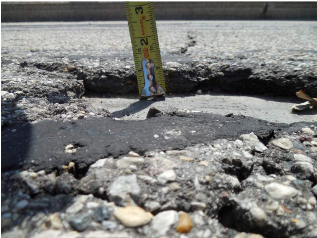
Photo illustrating thickness of asphalt, approximately 1 inch
