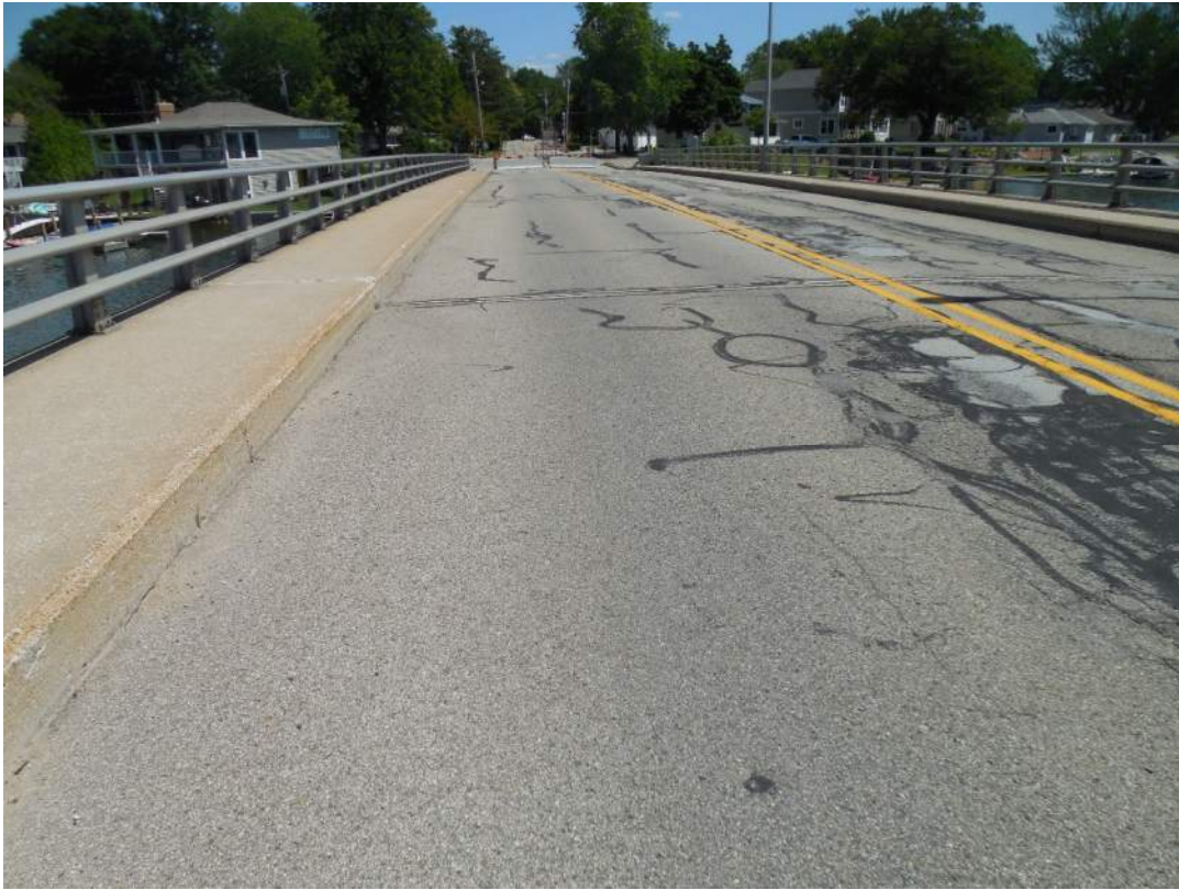
View of southbound lane, north half of structure, looking north
