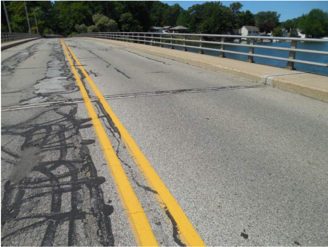
View of southbound lane near center of structure, looking southwest
