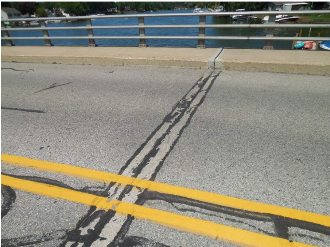
View of expansion joint in southbound lane, looking west
