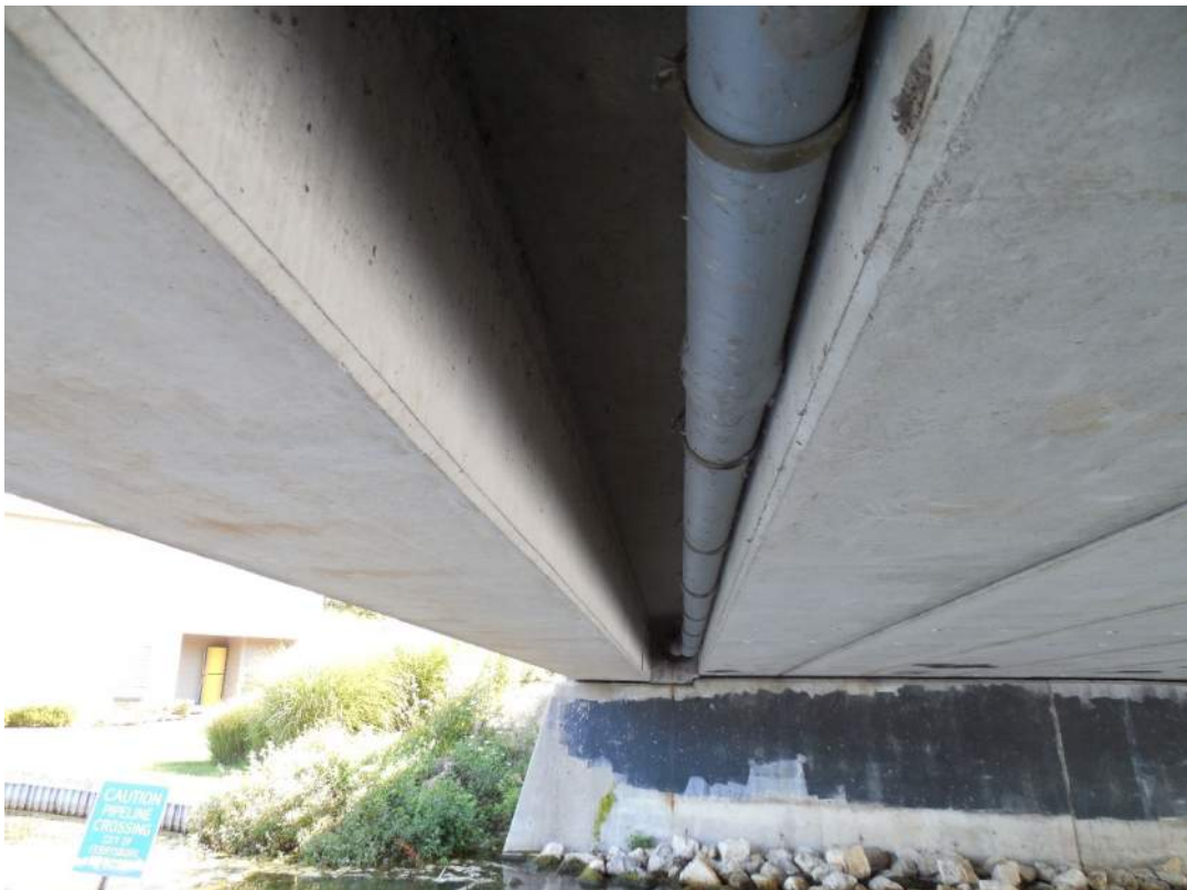
View of west utility chase, Span 8S
