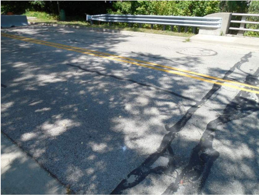
View of south approach pavement, looking southwest
