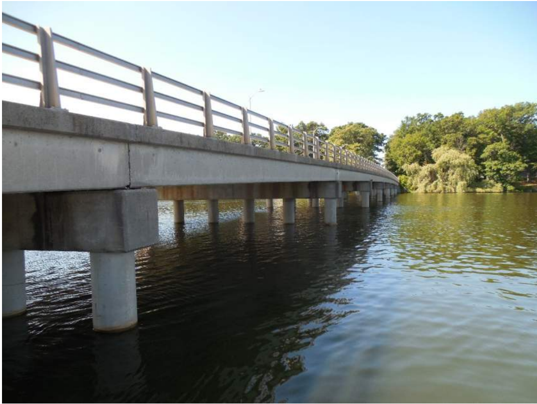
View of west elevation, looking southeast
