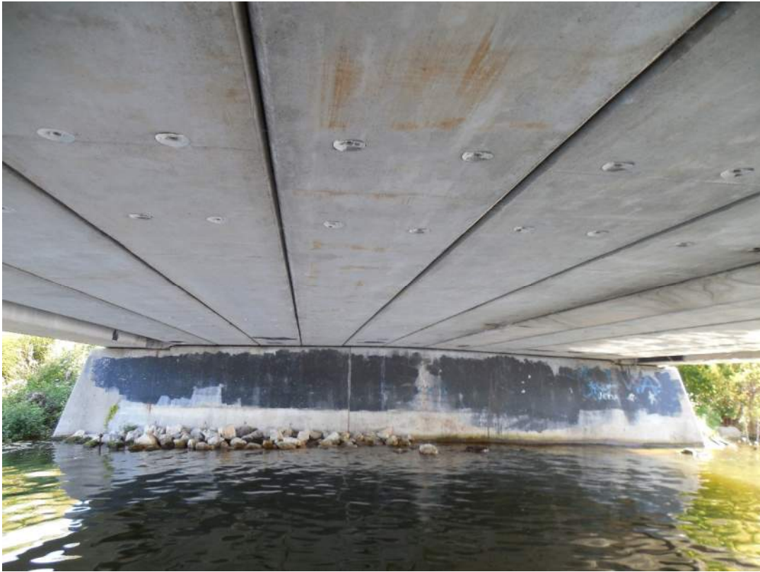
View of north abutment looking north
