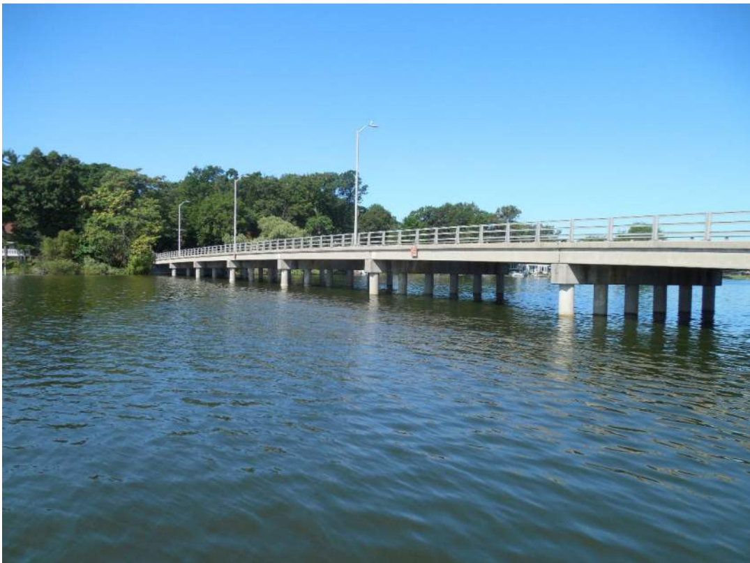
East elevation of structure looking southwest
