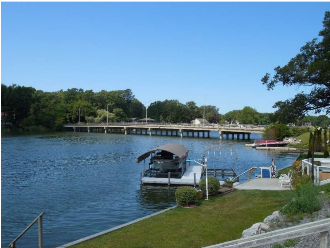
East elevation of structure, looking southwest from northeast shore
