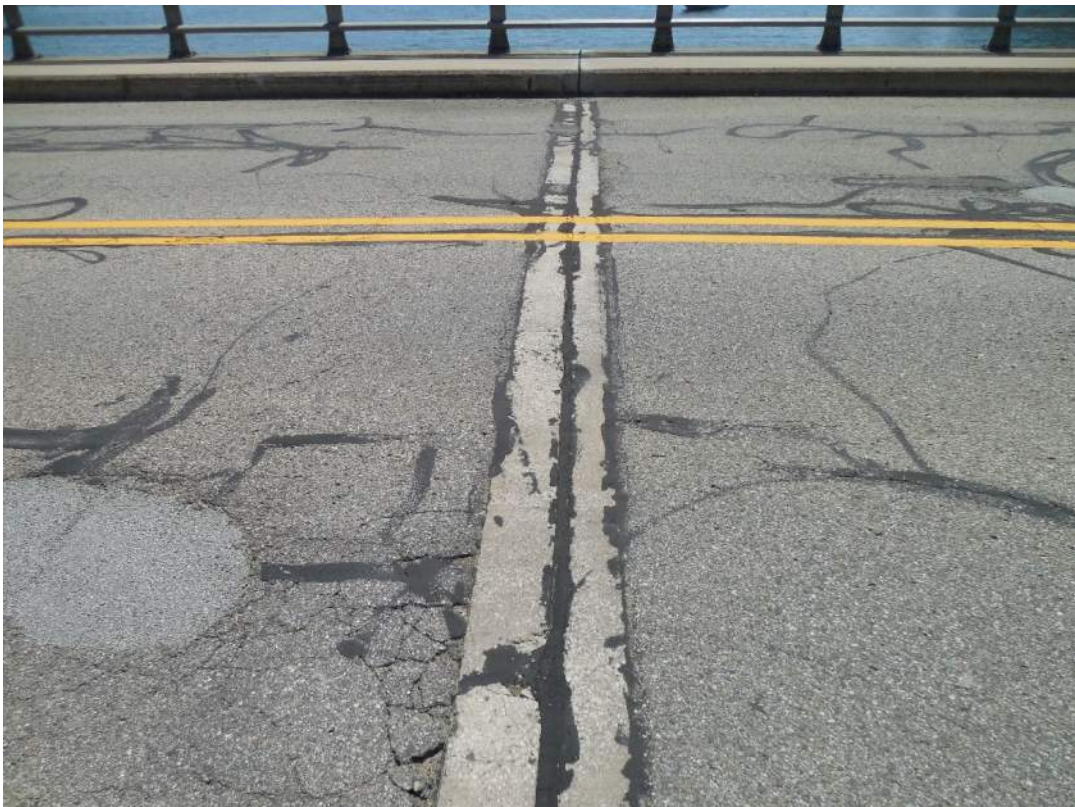
View of expansion joint looking east
